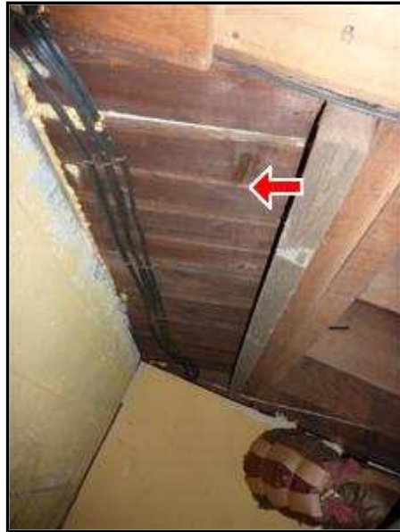
1.6 Picture 1 Wood forms under hearth extension
